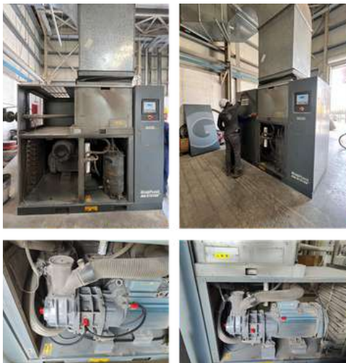
ATLAS COPCO compressor – 90 KV : 2 nos. installed with Intellivibe AI sensor
